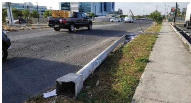
Figure 5. PR-506 downed pole near hospital in Coto Laurel.
