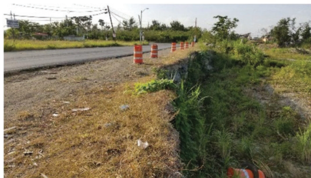
Figure 4. PR-511 Real Anon roadside damage.
